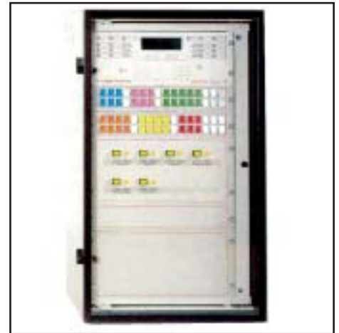
Fire alarm and control panel.
