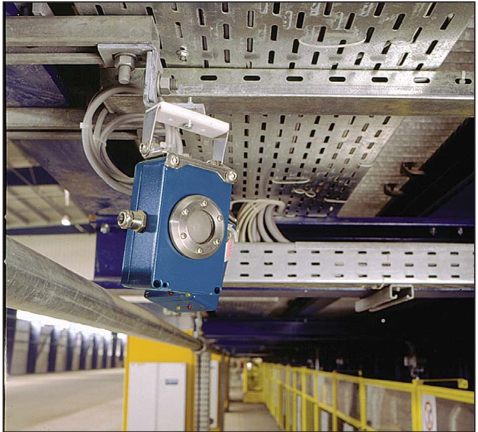
Flame Detector FMX 3511 with self-monitoring optic.
